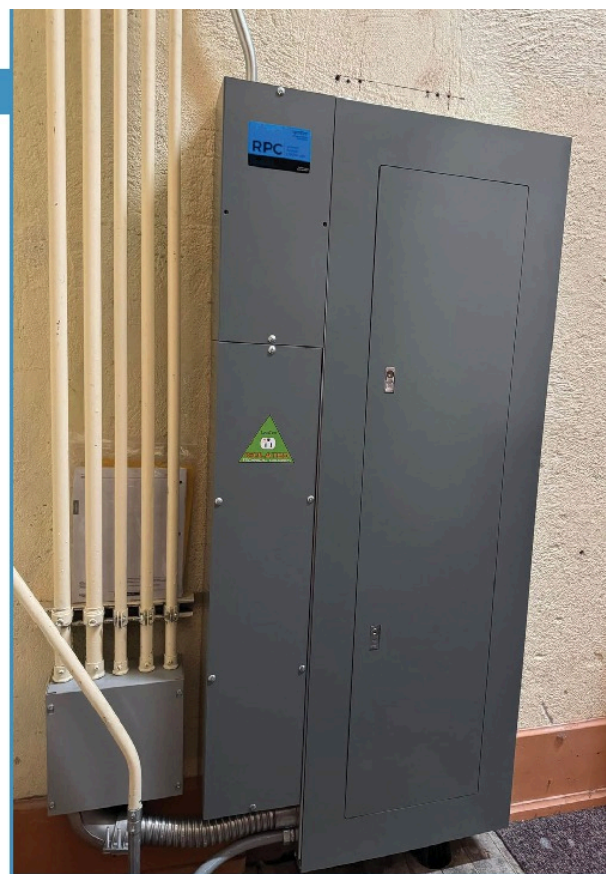
In the lighting upgrade, the existing 225A dimmer rack was replaced with a LynTec RPC 365, providing ample power and room for future expansion with 12 extra circuits.
